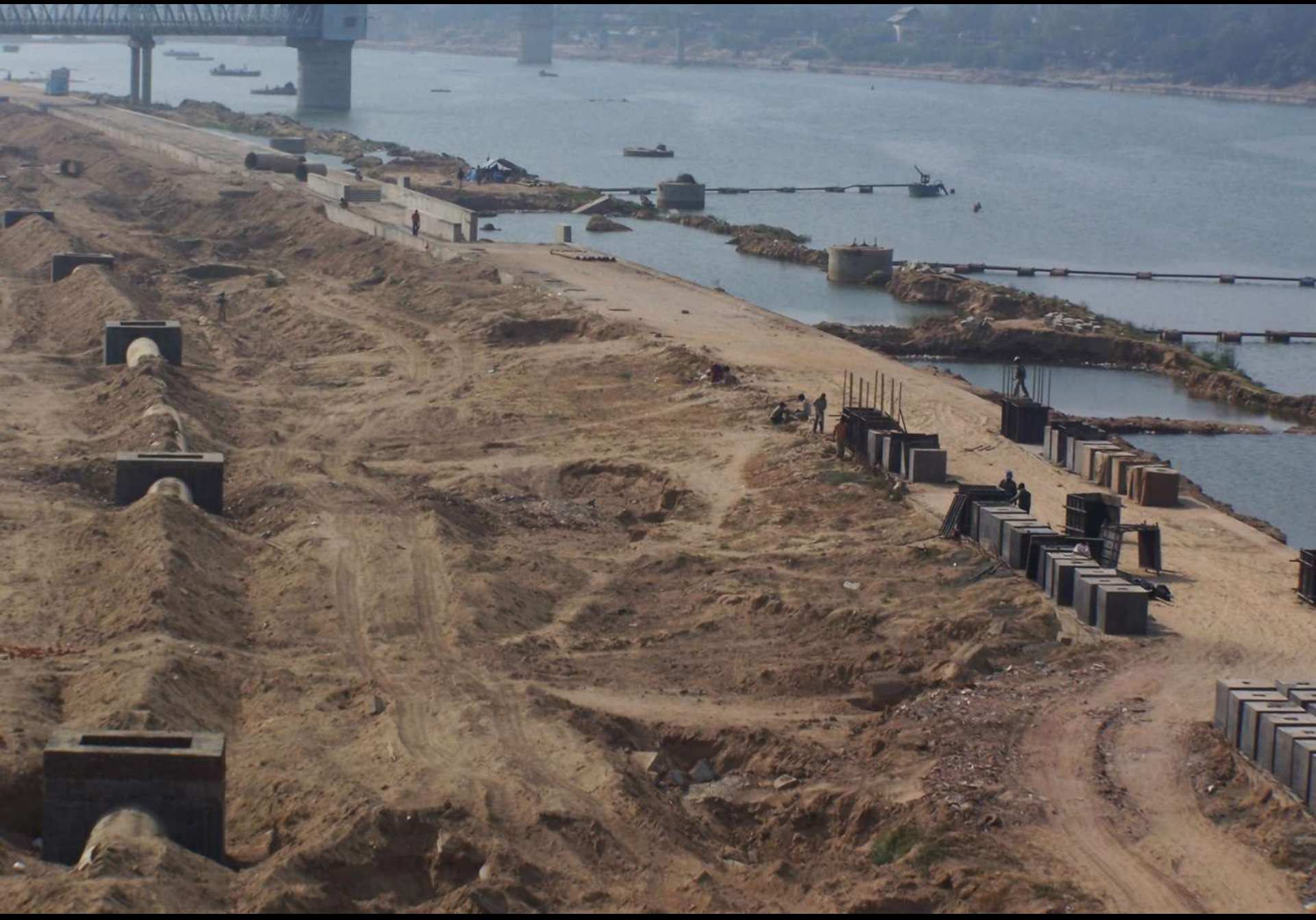
Interceptor sewage line being built
